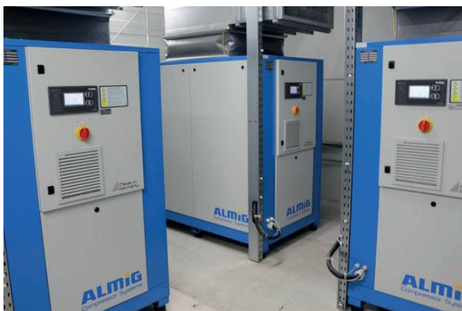
The powerful V-Drive series screw compressors: The energy-saving speed control achieves an excellent level of efficiency over the entire speed range.
