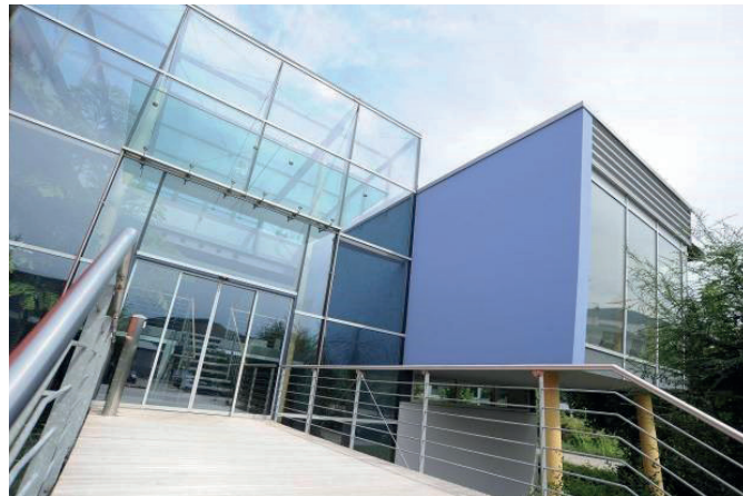
Creative and forward-looking solutions, the necessary technical know-how and custom-fitted production – Moser GmbH is on a growth trajectory. In its production, this manufacturer relies on screw compressors from ALMiG.
