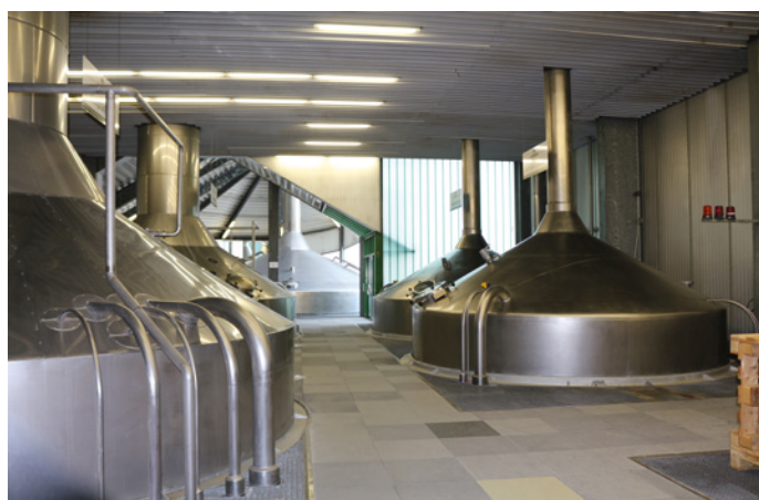
In the brewhouse, for example, the wort is ventilated with compressed air.
