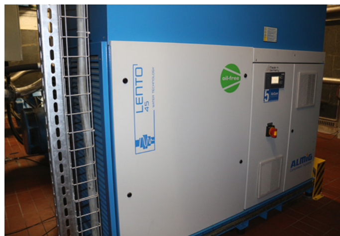
The oil-free, water-injected screw compressor from ALMiG not only ensures the Class 0 compressed air quality required in the beverage industry, but also an energy-efficient process technology.
