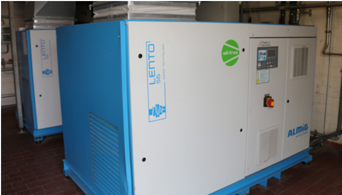
Bad Meinberger relies on oil-free water-injected screw compressors of the LENTO series from ALMiG.
