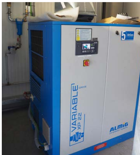
The Variable XP is used in low load phases - for example at night or on weekends.
