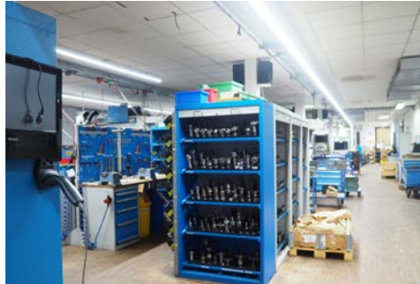
Compressed air is used almost everywhere in production.
