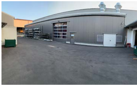
The new hall also houses the new compressed air station.
